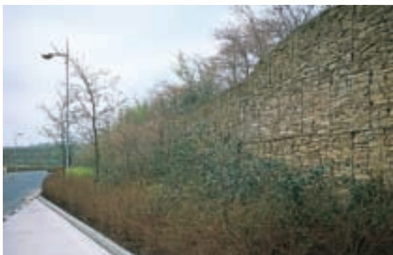
Gabion retaining wall using metal basket containing stone and rock.
