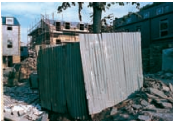
A poor example of tree protection. It is essential to safeguard trees during site works.
