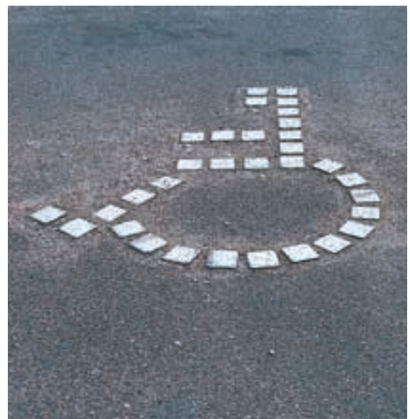
Example of a durable bay marking in granite setts.
